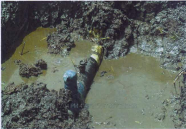
Figure 1: Installed Nipple on the pipeline.
